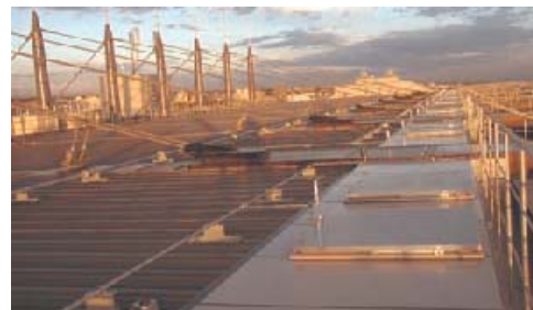
Figure 2: The roof of the stadium
